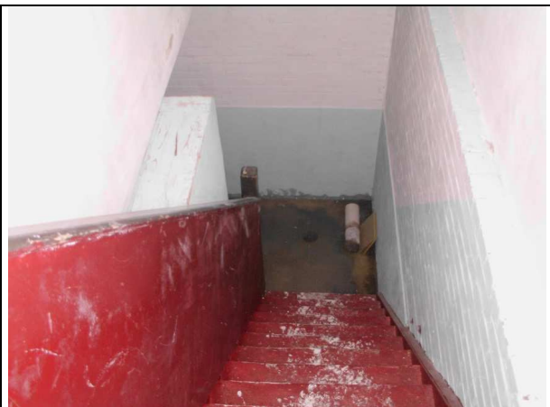
Trans 8 kelder, boring 16
