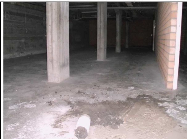
Trans 6 kelder, boring 18
